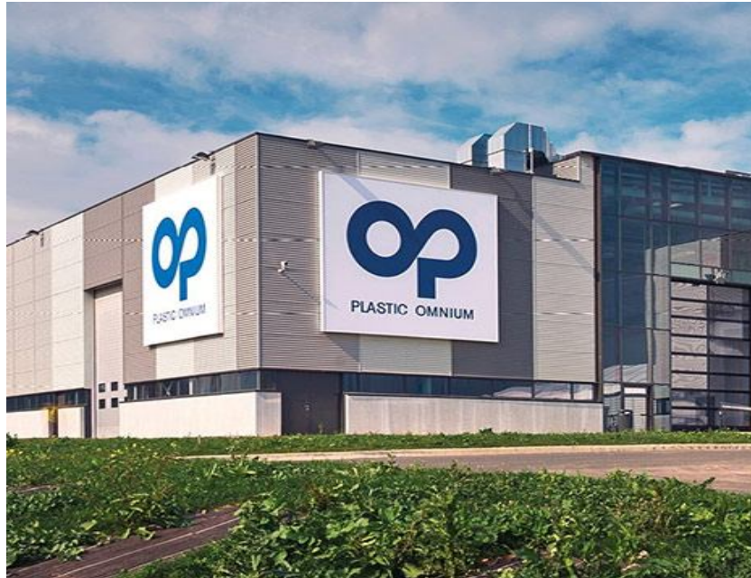
Project – Plastic Omnium Location – Gurgaon 3 units – UAL 450D5
